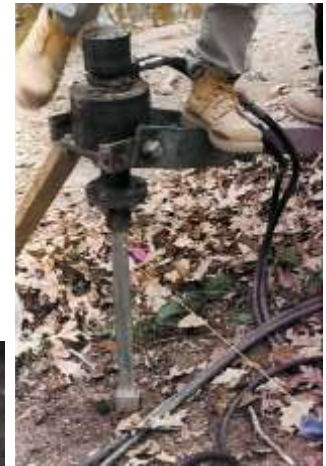
Helical pier installation
