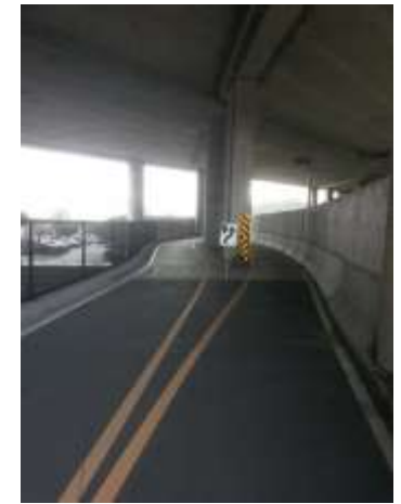
Trail tunnel with rail
