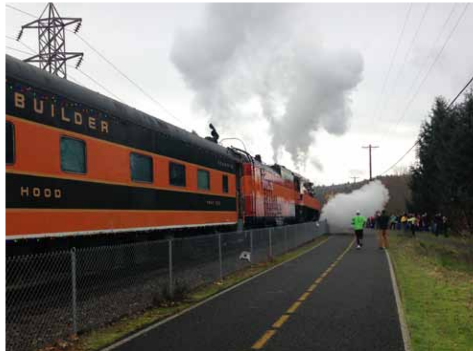
Springwater Corridor Rail With Trail, with safety fencing
