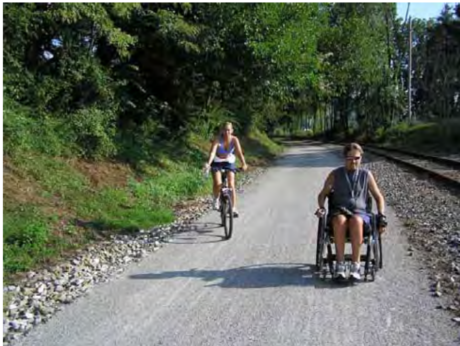
Rail With Trail using compacted aggregate for accessibility
