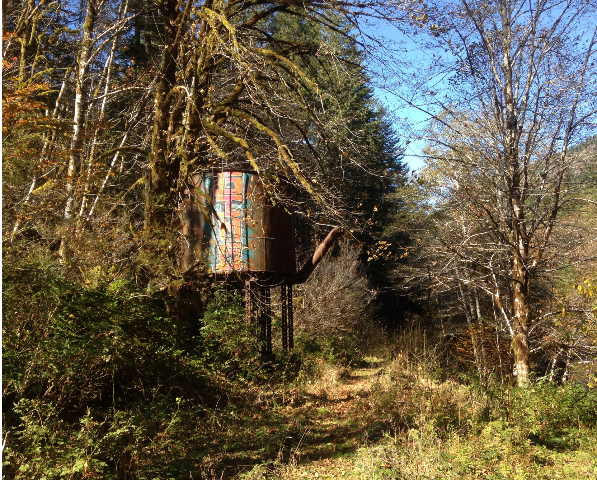
Disused railroad water tank, Milepost 811.25
